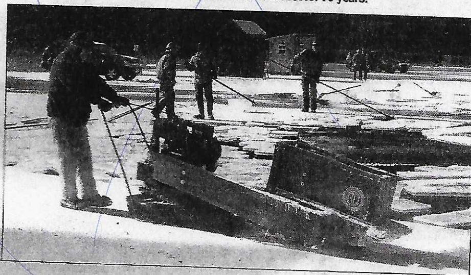
CARL HANSEN created the straight saw and is known as the sawyer in the process at the ice harvest.
